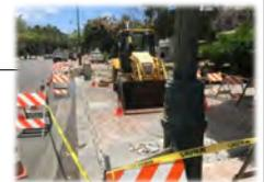
Mature tree roots had lifted the surface and pooling water was blocked from reaching the storm drain. One tree was removed and will be replaced with two, less mature trees in larger tree wells.
